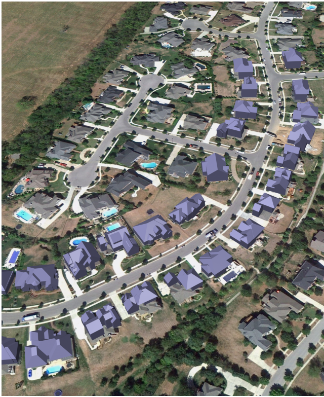
Figure 10: An overall view of reconstructed houses in Div-A.
